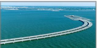
TheÖresund Bridge is a double-track railway and motorway bridge across the Øresund Straits between Scania (southernmost Sweden) and Denmark. The bridge runs nearly 8 kilometres (5 miles) from the Swedish coast to the artificial island of Peberholm, which lies in the middle of the Straits. The crossing of the Straits is completed by a 4 km (2.5-mile) underwater tunnel, called the Drogden Tunnel, from Peberholm to the Danish island of Amager. The term Øresund Bridge often includes this tunnel.
